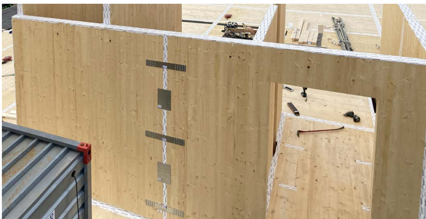
Example of CLT elements that are taped for protection during installation.
