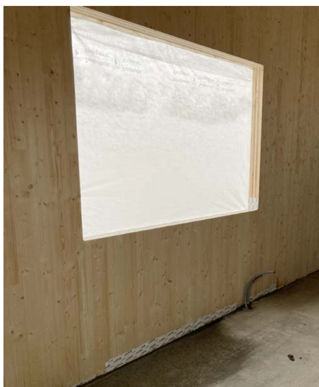
Weather-proofed window opening.
