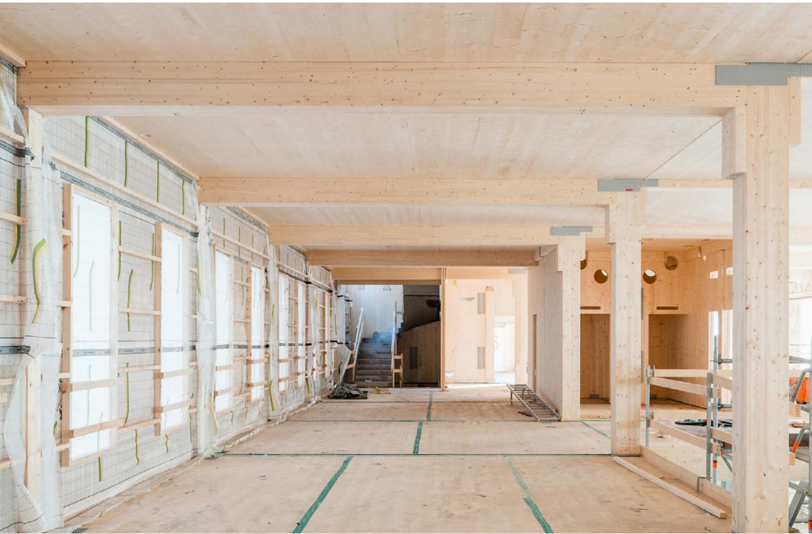
Ongoing CLT construction project.
