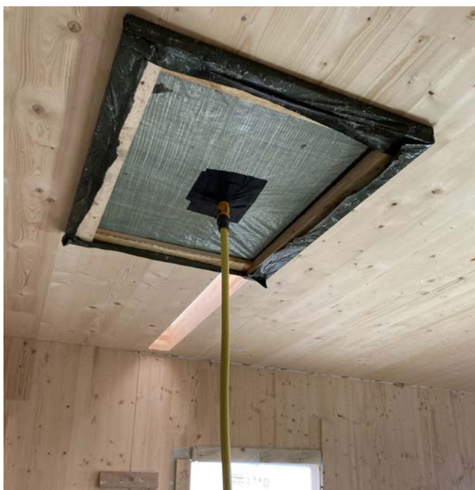
Example of temporary drain between floors.
