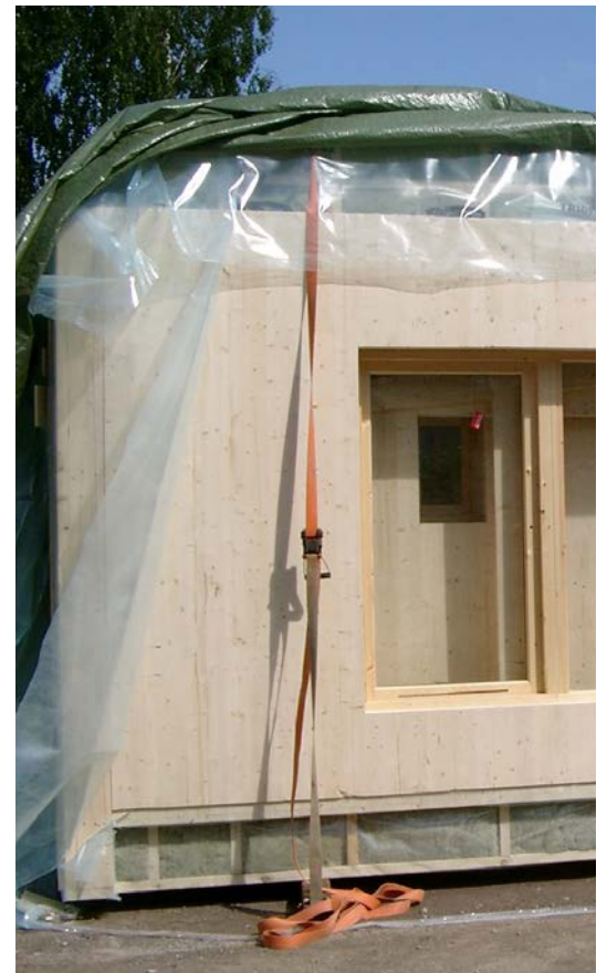
Prefabricated wall units being unwrapped for assembly
