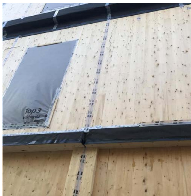
External wall with sealed floor edges and windows/doors.
