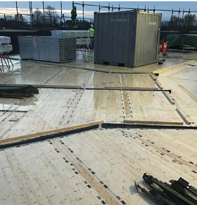
Floor system with taped joints.
