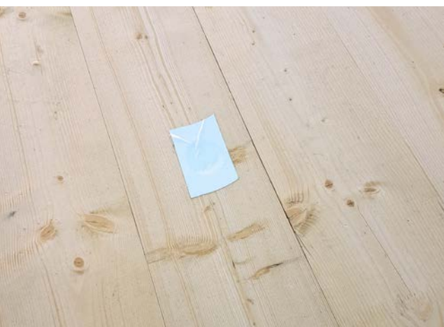
Sealing a small hole with tape.
